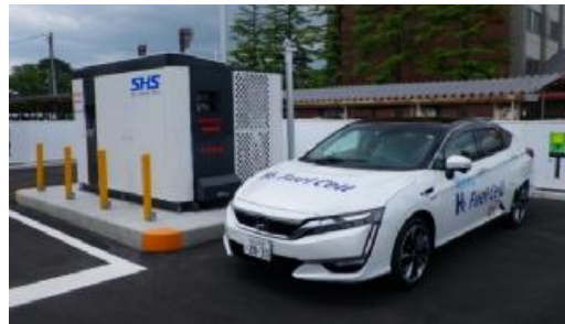
ü Operating Hydrogen Refueling Station and Fuel Cell Vehicle (FCV), toward a front-runner in using hydrogen as power source
