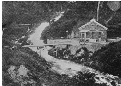
Numagami Hydroelectric Power Station, laid the foundation of Koriyama's development
