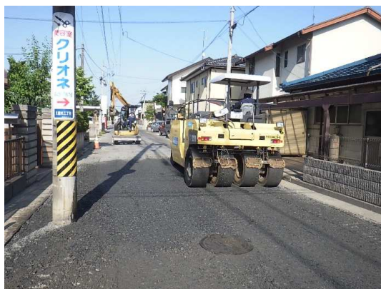
舗装仮復旧(路盤)状況
