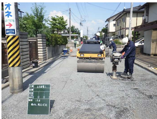
舗装仮復旧(路盤)状況
