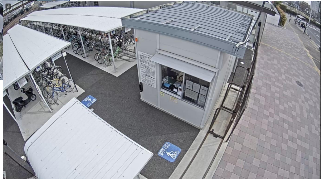
▼ Bicycle parking lot
