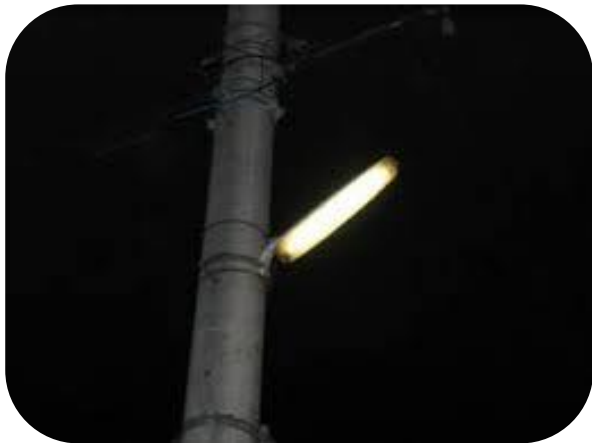
Previous fluorescent lights
